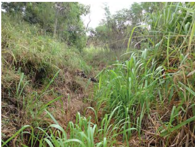
Photo 3: Paua Drainage Ditch
