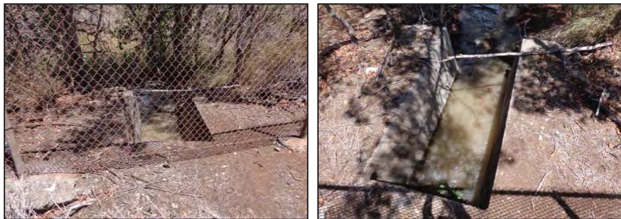
Photographs taken during tank flushing, following an inspection of the tank interior (August 2017)
