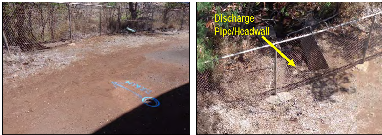
Photographs of the tank discharge pipe/headwall to the drainage ditch (August 2017)
