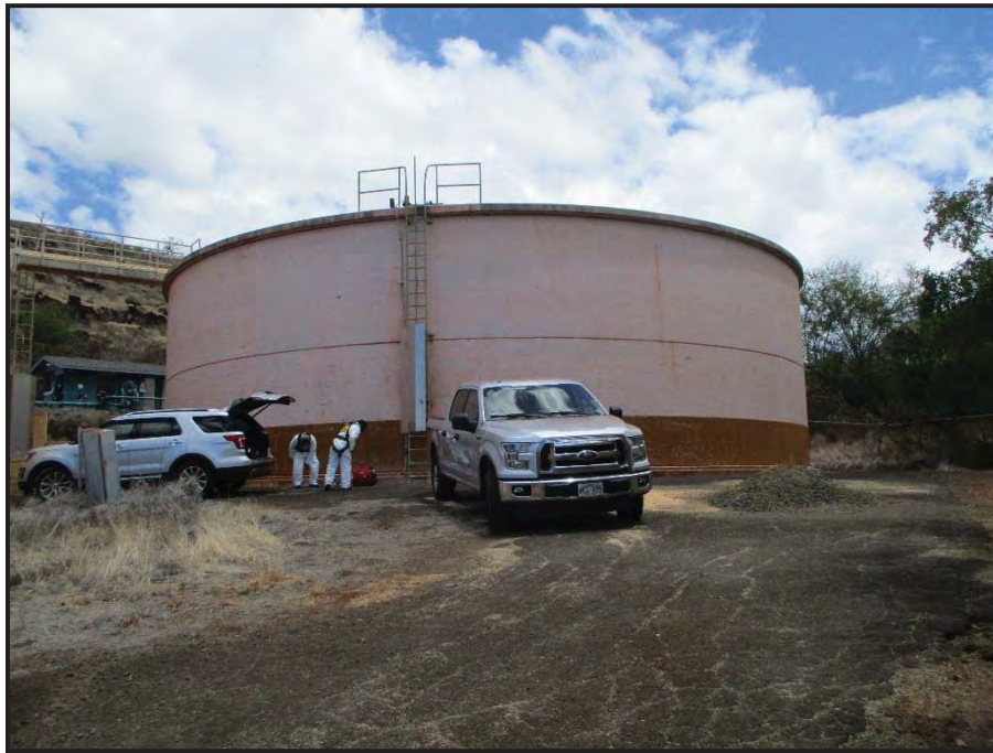
Kauai County DOW 0.5MG Tank August 2017
