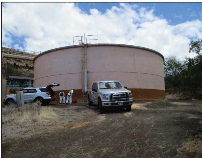
A View of Paua 0.5-MG Tank (August 2017)
