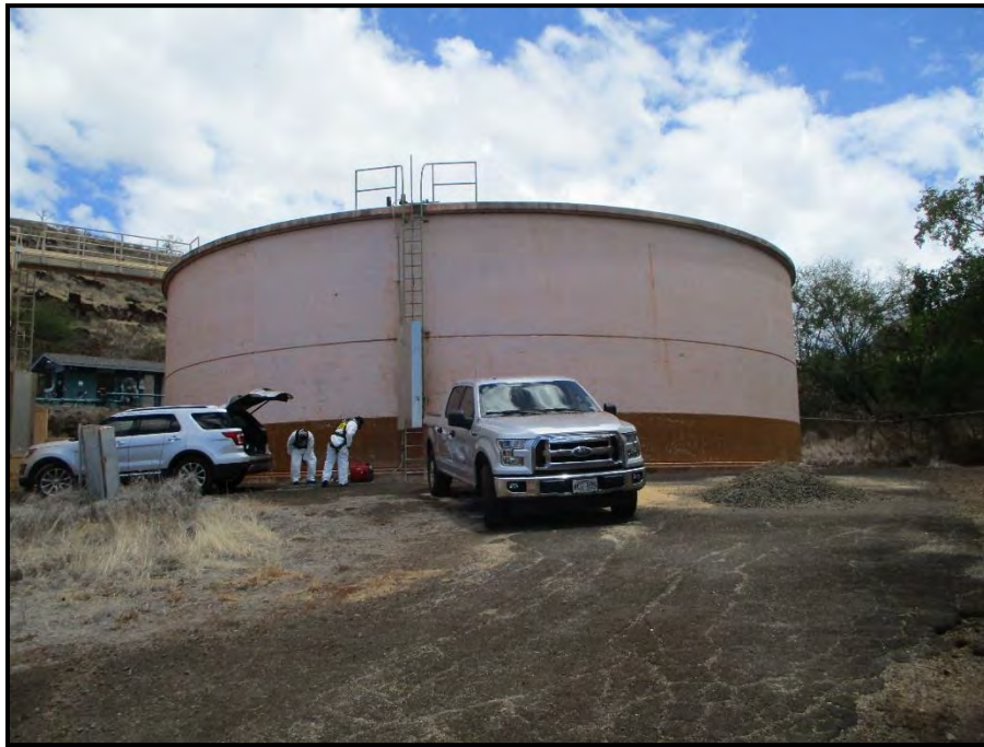
Kauai County DOW 0.5MG Tank August 2017
