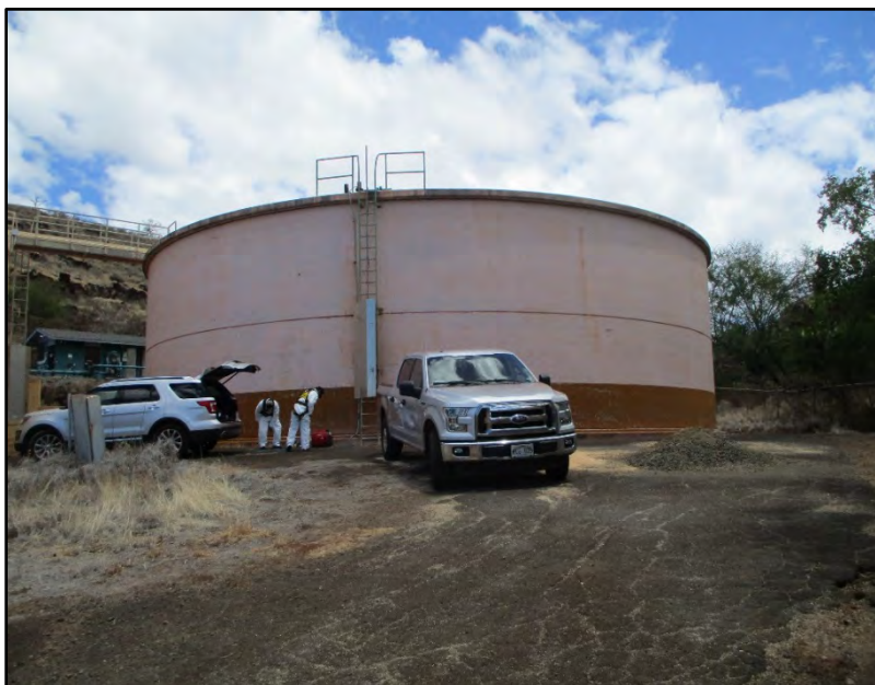
A View of Paua 0.5-MG Tank (August 2017)
